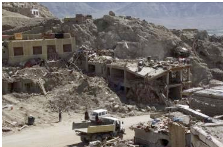
Fig. 1 – Leh, Ladakh: the destruction of the urban fabric after the heavy monsoon and related flood (credits: Désirée De Antoni, 2010)
